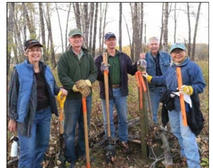
Post installation along Fish Creek, Oct. 9
