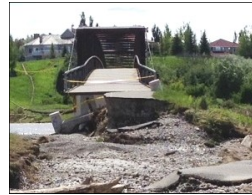
Bridge 14 near McKenzie, photo by Cheryl Arpin
