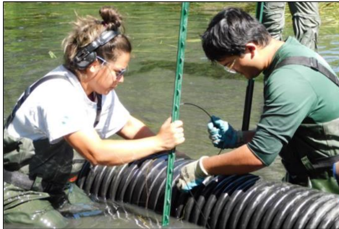
Himanshu Sangale, right, and a Wild Outside Participant securing the pipe on a new flow control device in the wetlands near Sikome Aquatic Facility, Aug 8. Photo, Rose Ratliffe
